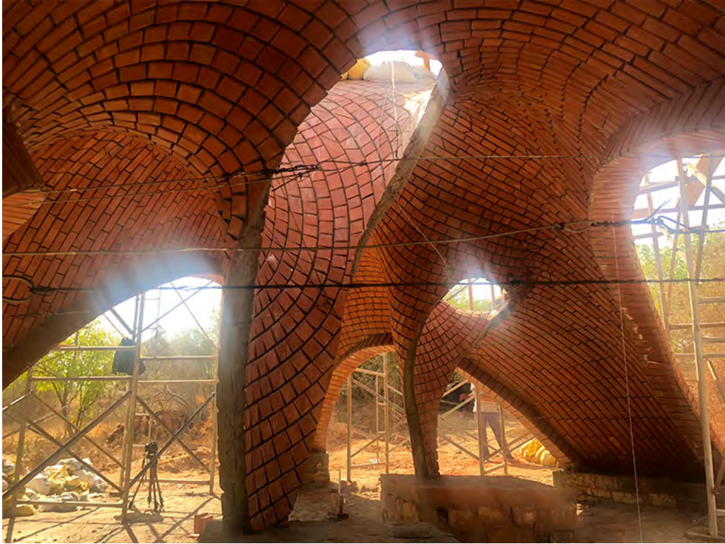
Figure 10 Prototype ready for load test
