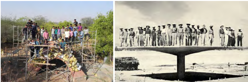
Figure 11 Physical load test similar to the thin concrete shell by Candela.
